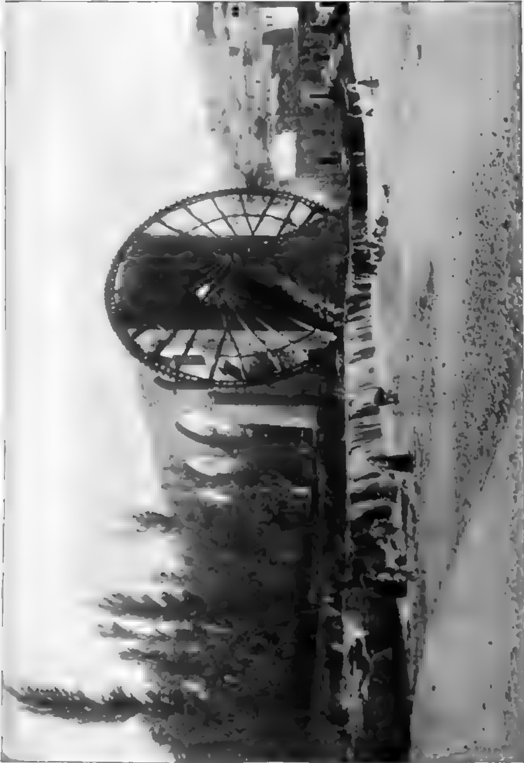
The great waterwheel at Hama, Syria, used for pumping the water out of the Orontes River
